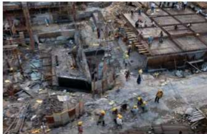
Fig 2-a typical view of a construction site
