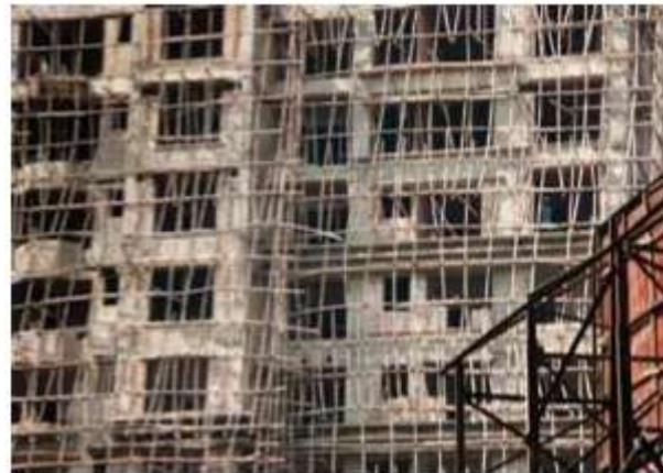
Fig 3-a typical view of scaffolding
