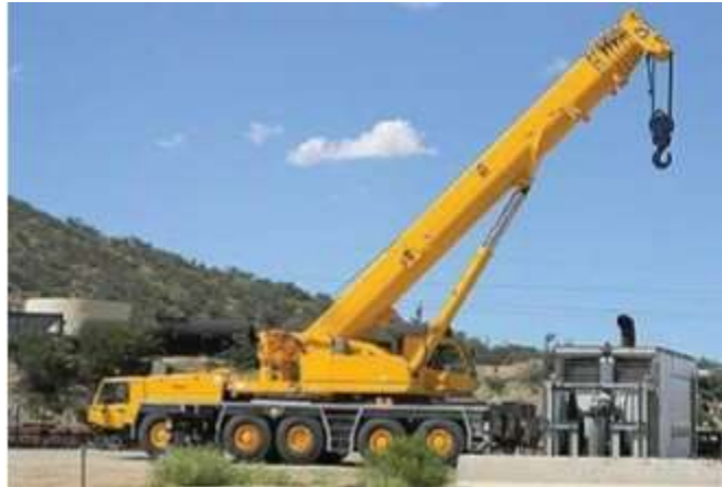
Fig-4 Demonstration of a typical mobile crane in operation
