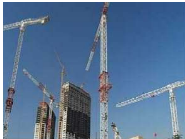
Fig-5 a typical view of tower cranes
